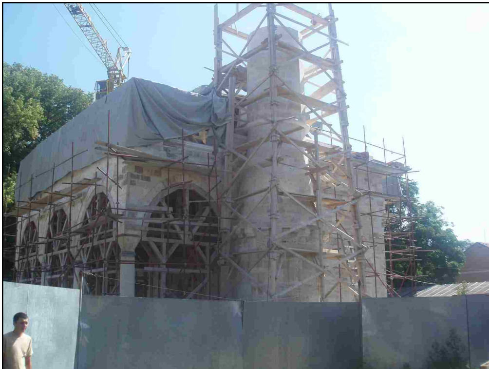
Figure 2.25: Photograph from approximately the same vantage point as Figure 23 but in August 2011. The project team anticipates finishing the construction in one year. Image by author.
