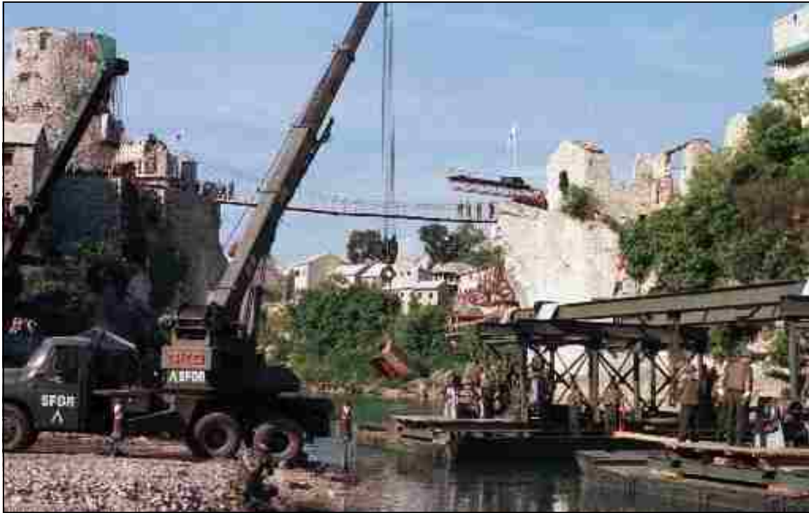
Figure 2.12: Hungarian SFOR engineers lift stones from the Stari Most out of the Neretva River on Monday Sept. 29, 1997. Photograph from AP Photo/Jozo Pavkovic.
