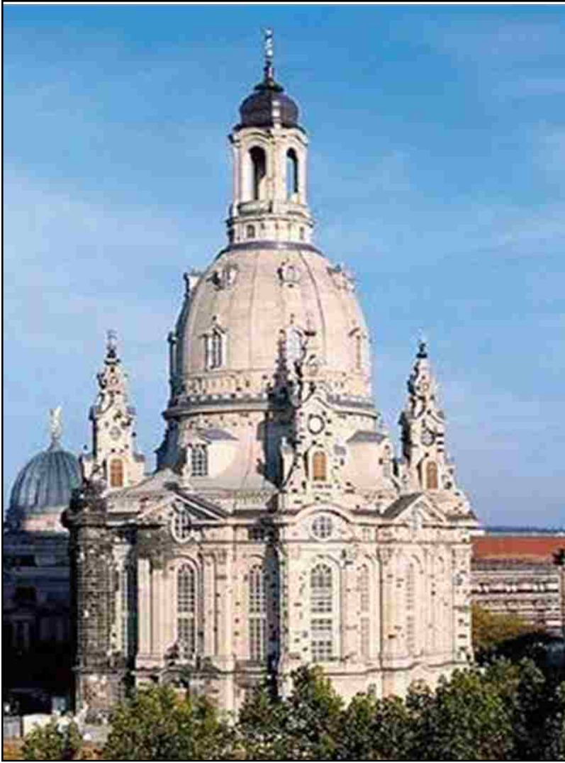
Figure 2.9: The reconstructed Frauenkirche with darker, original stones visible in the lower, left hand corner of the structure. Image from Frauenkirche website.
