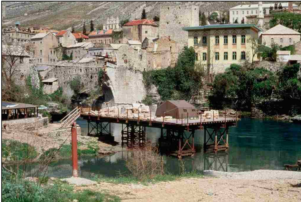
Figure 13: Photograph of the staging for the salvage and reconstruction of Stari Most in 1998. Photography by Jon Calame.
