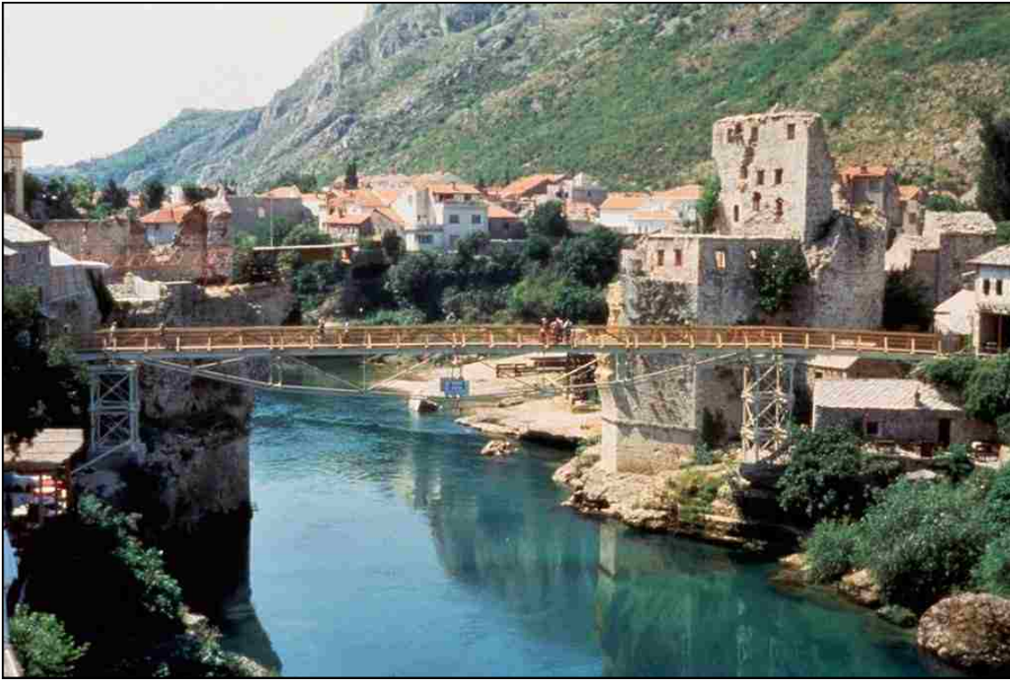
Figure 2.14: Temporary bridge over the Neretva River prior to the reconstruction. Additionally, damage to the buildings along the river is visible in the photograph. Photograph by Jon Calame.
